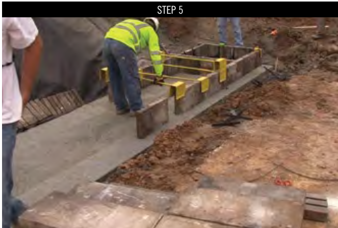
Start the Mega-Tandem™ (MSRW) at the lowest elevation. Start by setting the panels in place with the use of the wall jigs to help support the panels during the wall installation.
