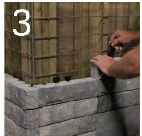
Attach Tandem Veneer with Connector
